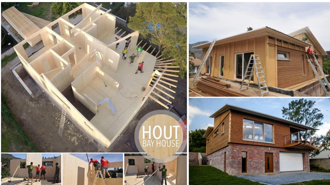
Figure 1: Hout Bay House and its construction
